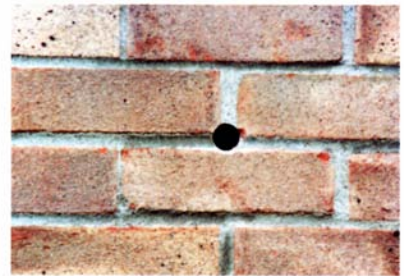
Neat hole ready to receive fill
