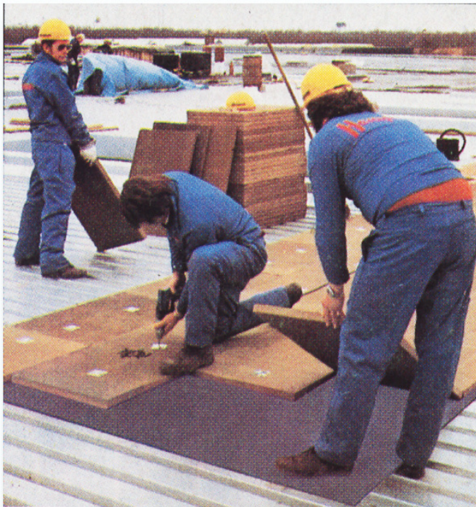
Workers installing Rockwool Concrete Board over waterproofing material
