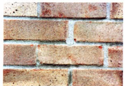
Hole sealed with mortar
