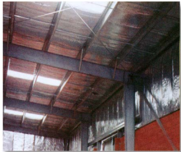
Metal Structure Insulation with Aluminum Facing used as roof and wall insulation
