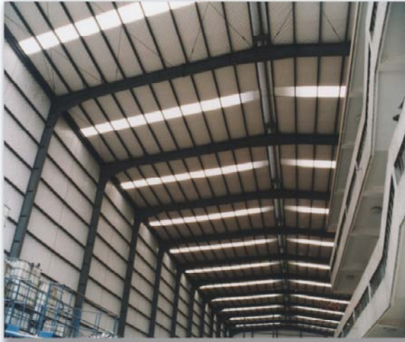
Metal Structure Insulation with Vinyl Facing used as roof and wall insulation
