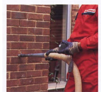
Blown wool being injected
